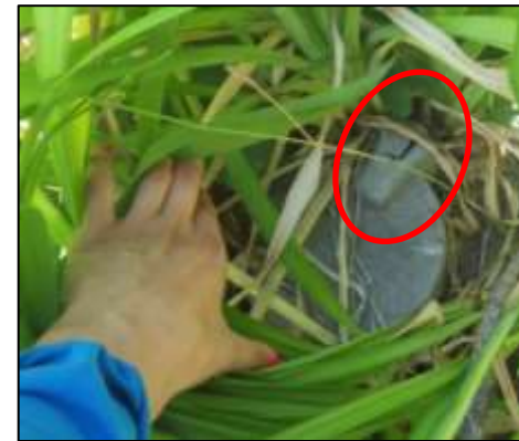
Well casing surrounded by day lilies and showing damage to the cap
